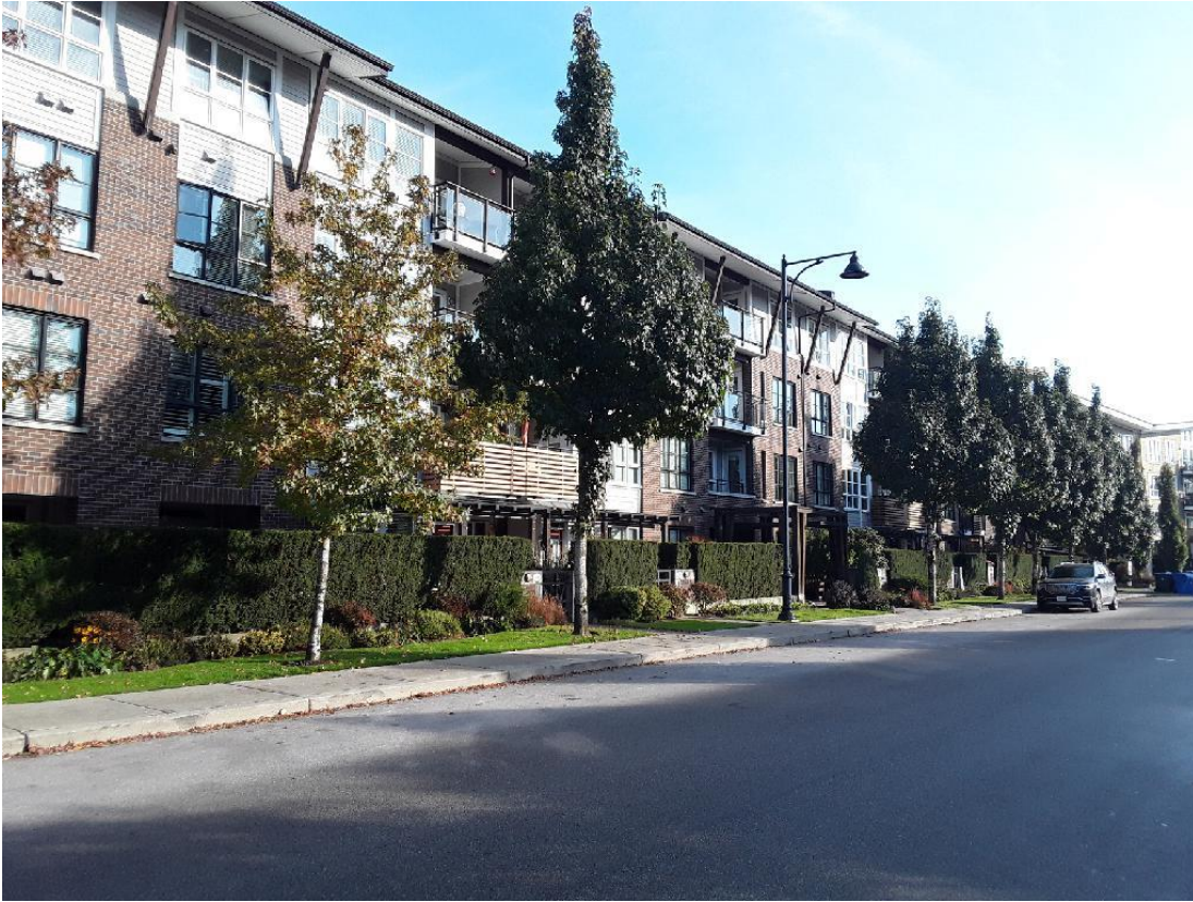
Figure 7: Newly completed apartment complex with highly flammable cedar hedging planted.
