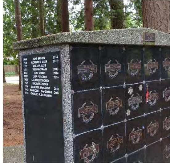
Figure 8: Columbarium Niches, Source: LEES+Associates.
