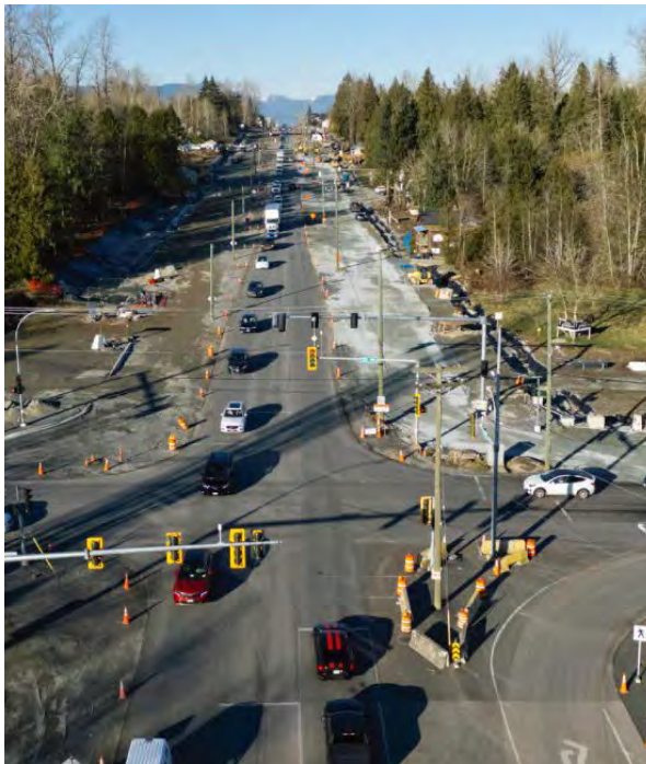
Construction progresses on 208 Street and other roadways
